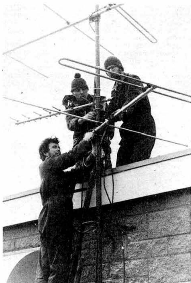
New 70 and 144MHz antennas being fitted at the GB3ANG beacon installation. Up the pole and on the tiles are, l to r: Chris Tran, GM3WOJ; Peter Bates, GM4BYF; and Malcolm Hamilton, GM3TAL. Photo: G3UUT
